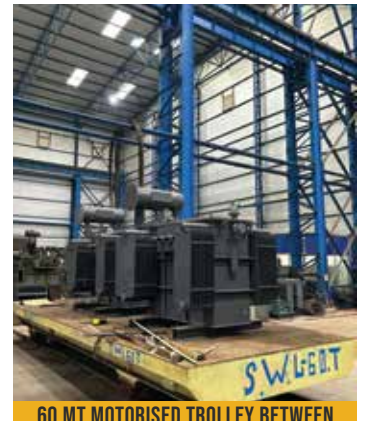
60 MT MOTORISED TROLLEY BETWEEN MANUFACTURING BAY'S
